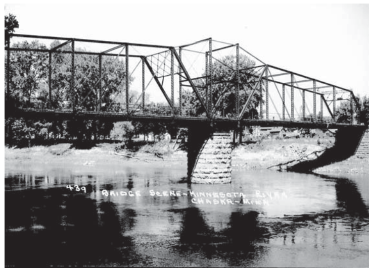
Historic truss bridge on Highway 41
