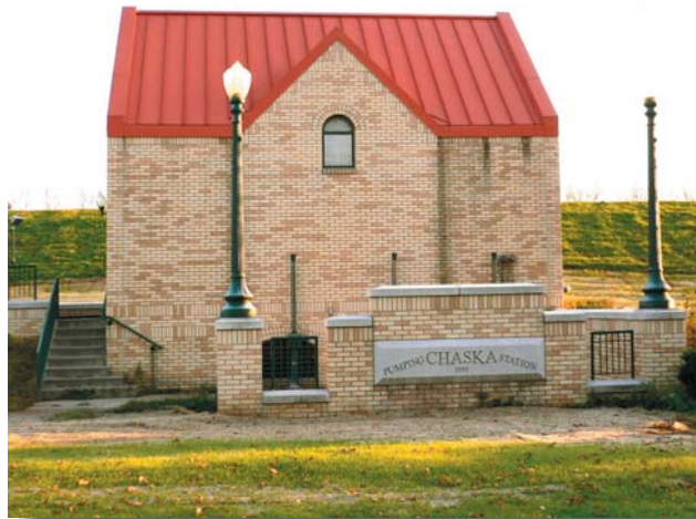
Pumping Station constructed in 1995
