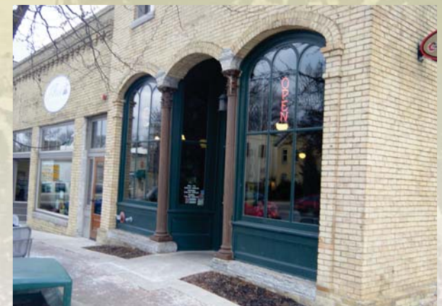
Restoration of the Philip Henk historic building on Second Street East added a full window storefront at street level with offices above
